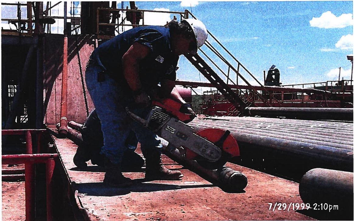
Photograph 13 - Lake Meredith Salinity Control Project: A subcontractor is cutting the inner barrel and core into sections. The core was from the 2155 to 2185 ft interval in Injection Well No. 1. Both ends of each barrel section are sealed, and the core is then transported to a core laboratory for testing. Photographed 7/29/1999 by Dennis McDonough.
