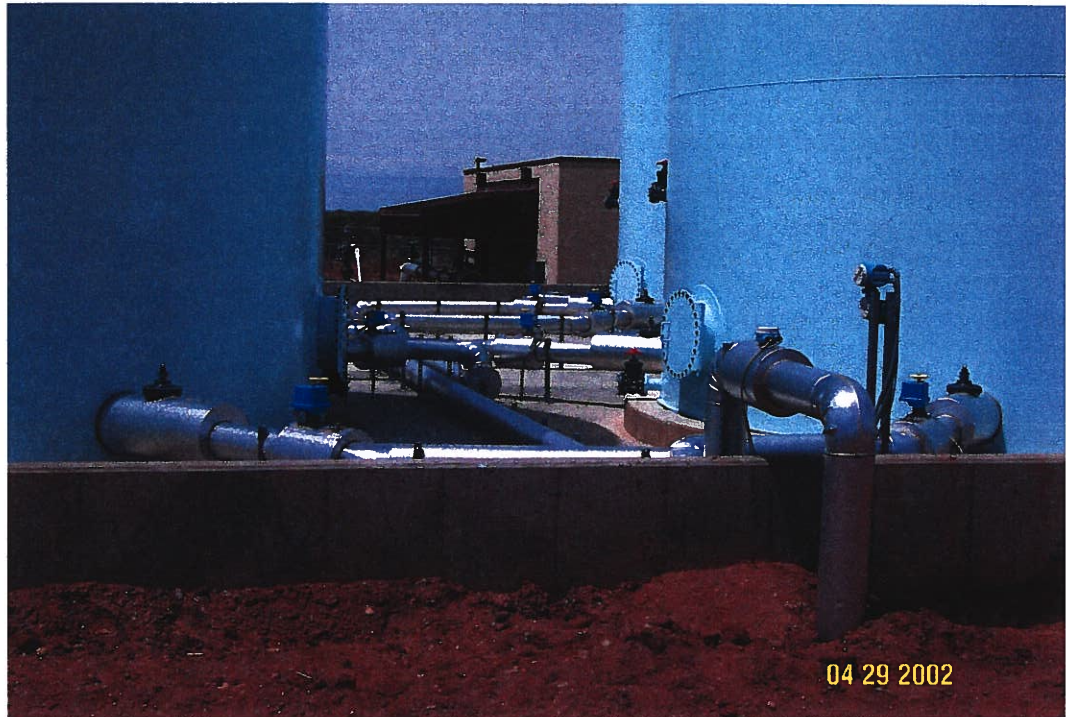
Photograph 44 – Lake Meredith Salinity Control Project: Pipeline from production wells enters the containment structure and storage tanks. The injection building is in the background. Photographed 4/29/2002 by Dennis McDonough.
