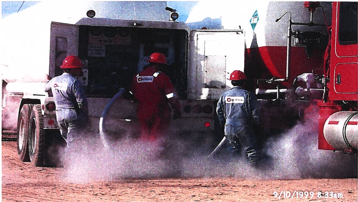
Photograph 17 – Lake Meredith Salinity Control Project: A Halliburton crew is performing nitrogen back-flow (lift) to stimulate the injection well. Photographed 9/10/1999 by Dennis McDonough.
