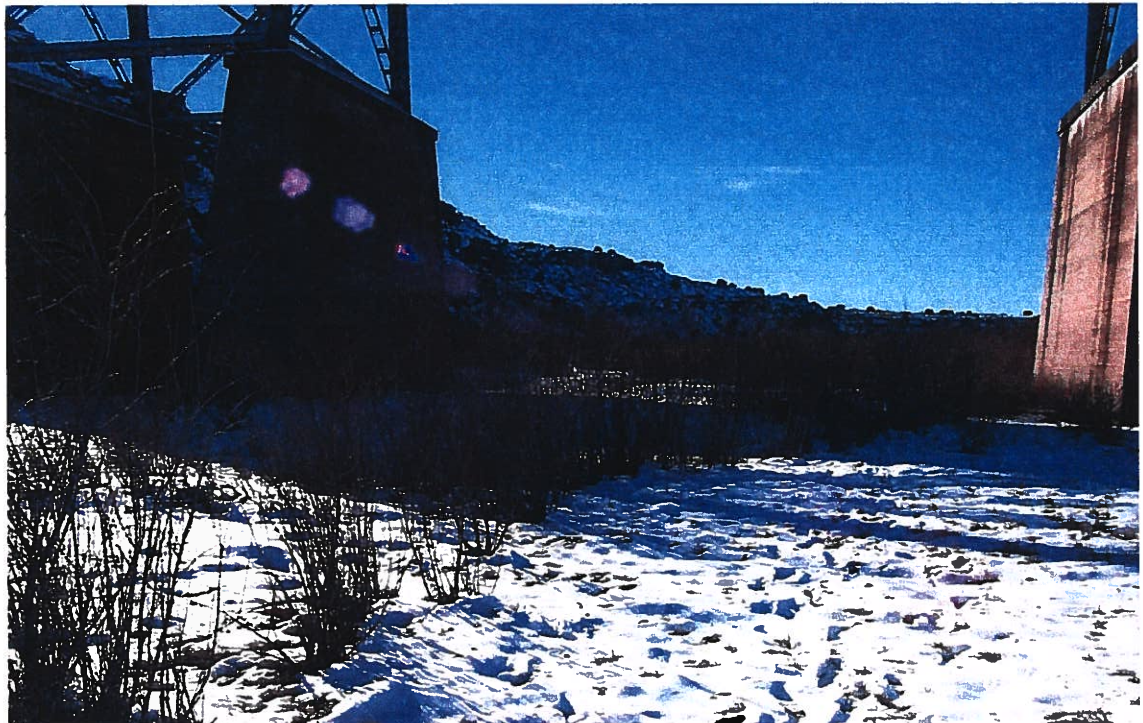
Photograph 28 – Lake Meredith Salinity Control Project: Looking upstream towards the west, the staked East Branch Pipeline alignment ran from the middle foreground through the extreme upstream corner of the concrete bridge footing in the left middle of the photograph. The alignment was revised to run the pipeline centered and parallel between these two footings. Photographed 1/3/2001 by Dennis McDonough.
