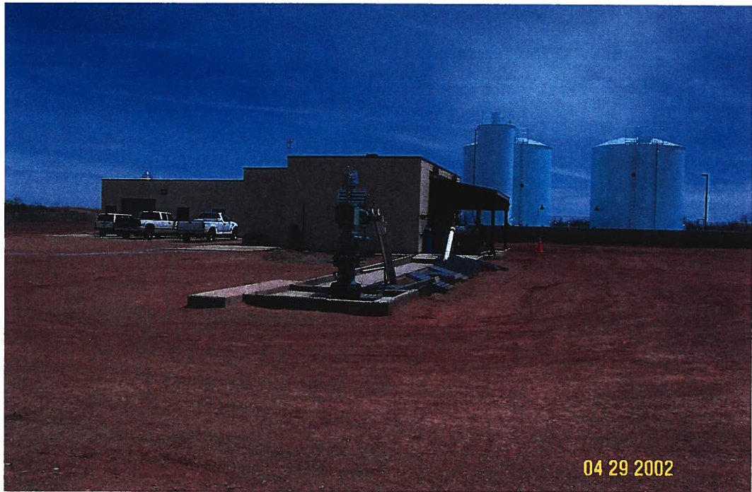
Photograph 50 – Lake Meredith Salinity Control Project: This view of the injection well facilities is to the northeast with injection well IW-1 in the middle foreground. CRMWA Corp. employees have added curbs to the well chase to prevent debris from entering. The gratings have been removed from the discharge line (well chase) from the injection pump. The injection pump and injection building are directly behind the injection well. The containment basin and storage tanks are to the right, and the office building is to the left. Photographed 4/29/2002 by Dennis McDonough.
