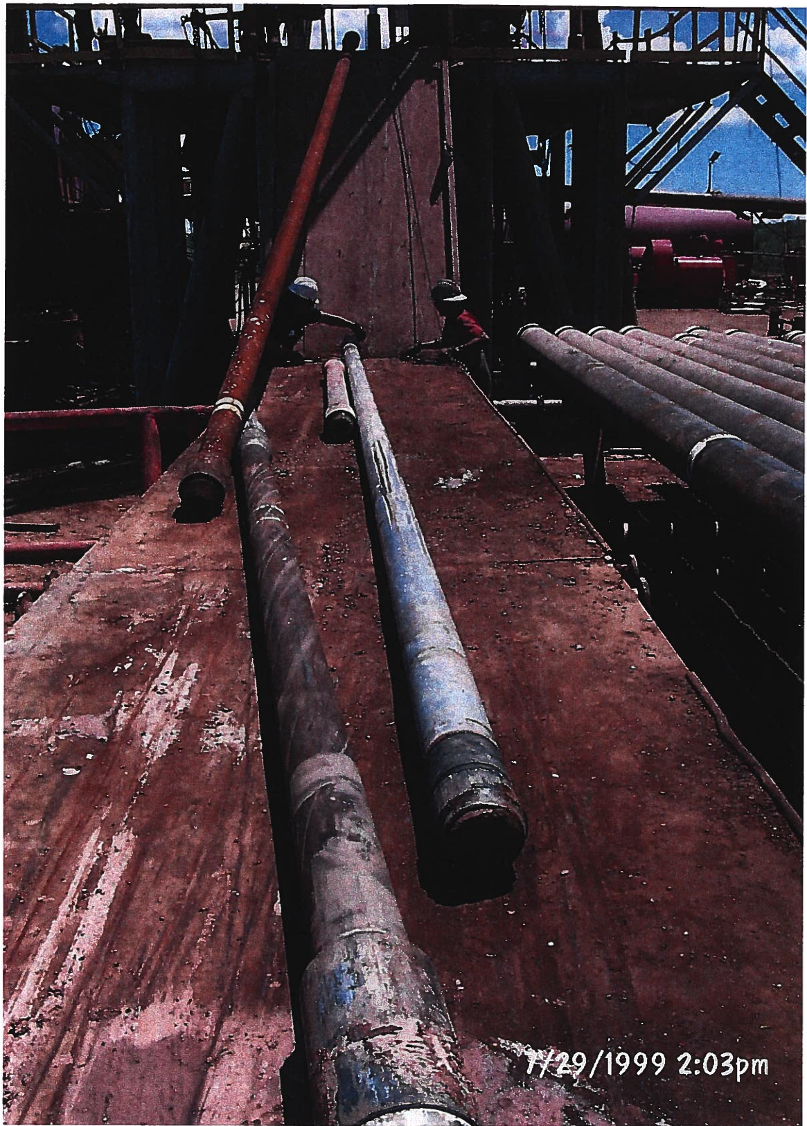
Photograph 12 – Lake Meredith Salinity Control Project: The inner barrel with inner barrel shoe has been placed on the platform. The exposed bottom end of the core is from cored interval 2155 to 2185 ft in Injection Well No. 1. Core recovery in this 30 ft run was approximately 26.0 ft. Photographed 7/29/1999 by Dennis McDonough.
