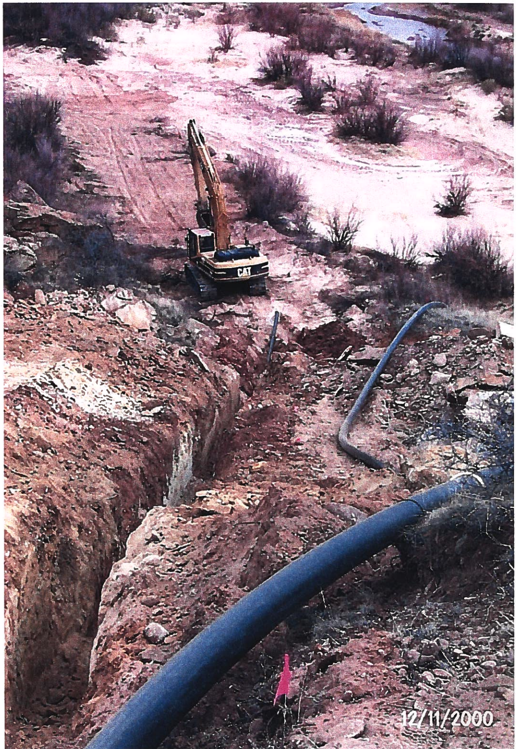
Photograph 29 – Lake Meredith Salinity Control Project: The Cat trackhoe has just finished excavating the West Branch Pipeline from plateau down the canyon wall to the Canadian River valley floor. Production Well PW1-1 is at extreme upper left. The trackhoe will travel back to plateau edge and begin laying bedding from the top down before the 6-inch diameter welded HDPE pipe is placed in the trench. Photographed 12/11/2000 by Dennis McDonough.
